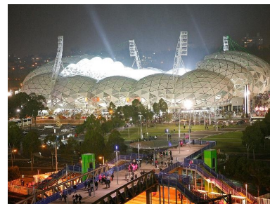
AAMI football stadium
