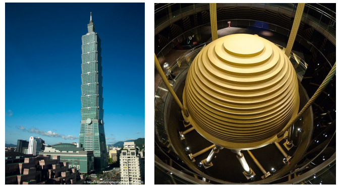
The Taipei 101 skyscraper and the damping pendulum inside
